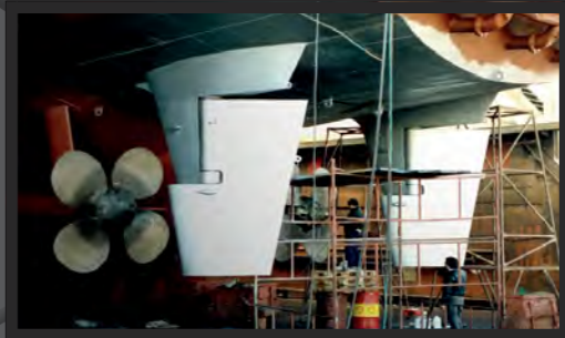
Construction and installation of rudders
